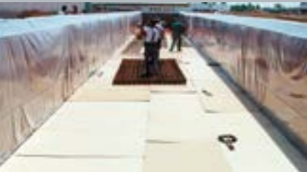
Figure 3: Block preparation for pouring the foundation
