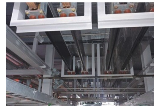
Cu bus bar 20T x 350W x Max 5000mm
