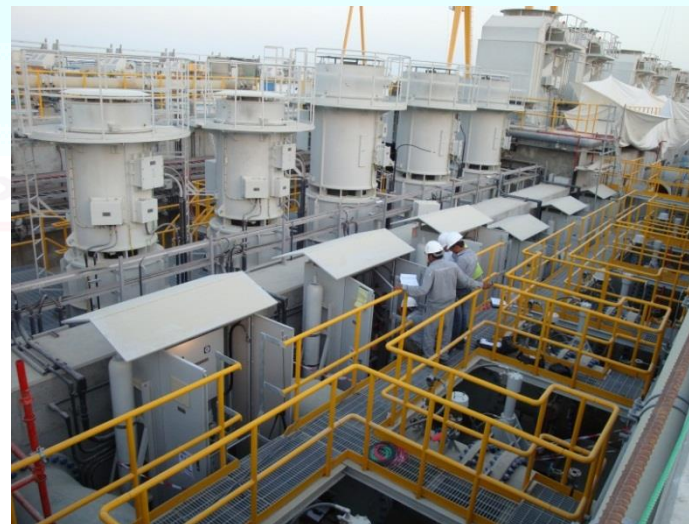
► MARAFIQ POWER & DES. PROJECT - Hyundai Heavy Industry - DN 1950
