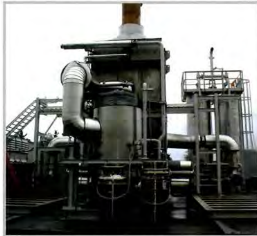
Fuel Humidifier (POSCO Power)
