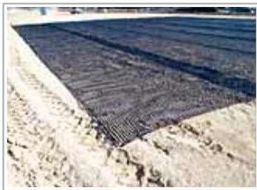
Reinforcing weak foundation
