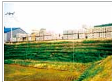
Reinforcing soil slop
