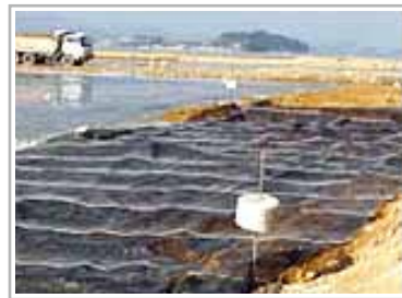
Stabilizing ultra soft ground
