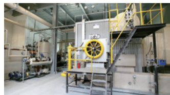
Tube Type Steam Boiler (20 ton/hr x 20kg/cm 2 )
