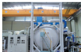
Tube Type Steam Boiler (20 ton/hr x 20kg/cm 2 )
