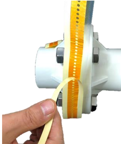
Step 2. Remove the release liner
