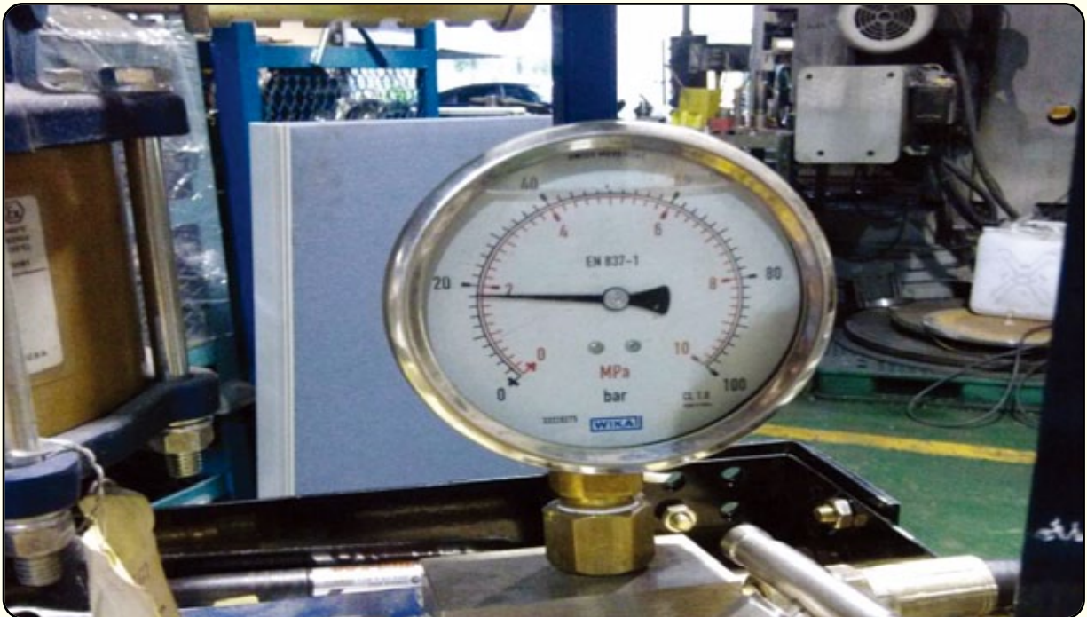
Photograph Explanation: Welding Type Butterfly Valve sheet leak inspection
