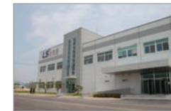
Tractor Engine Plant
