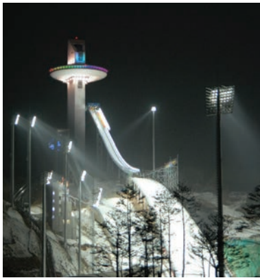
ALPENIA SKI JUMPING TOWER / CINDI SYSTEM
