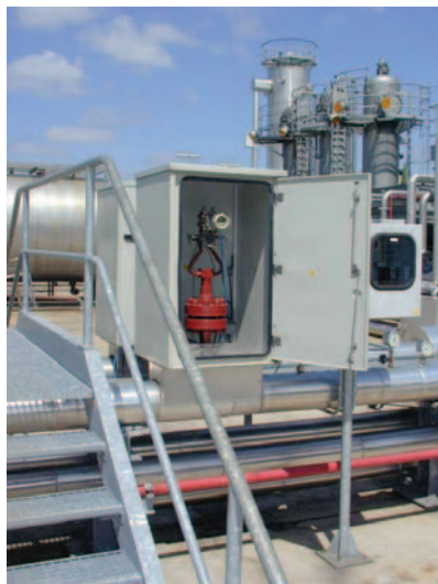
DF25HDD3 for polluted, high-pressure natural gas behind a drill head.
