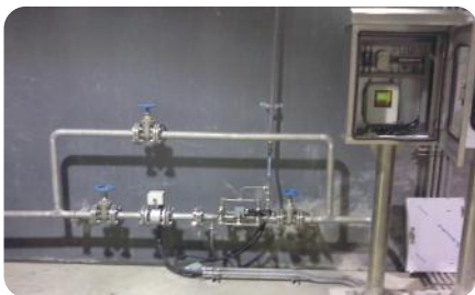
Munoseong Disposal Plant of Sewage
