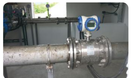
Ssangchi Disposal Plant of Sewage
