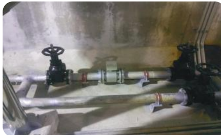
Gyeongsan Disposal Plant of Sewage
