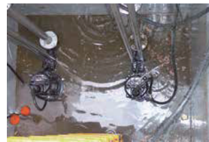
GRINDER PUMP INSTALLATION
