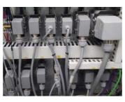
All cable connectors to controllers are located inside the stainless cage provide complete protection for electronic system from water and dust.
