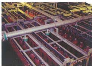
▲ Main Pipe Assembly
