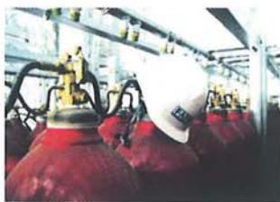
▲ CO2 Cylinder Assembly
