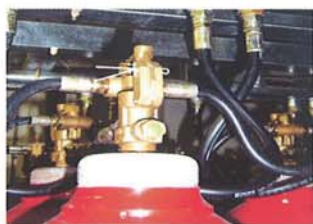
▲ Cylinder Valve Assembly
