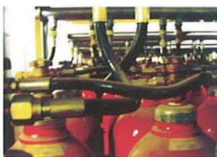
▲ Pilot & Flexible Hose Assembly
