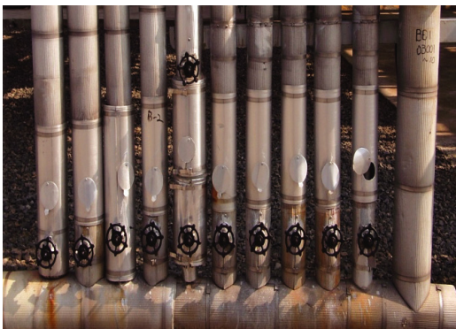
Piping & Field Insulation
