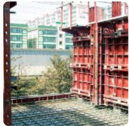
● SYSTEM FORM 적용 MOCK-UP TEST
