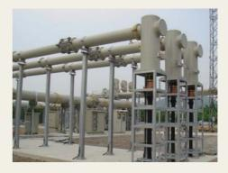
They also use epoxy insulating plate to isolate between cable sheath and GIS chamber. The SVLs(Sheath Voltage Limiter) can be installed to protect epoxy insulating plate from switching impulse. Upon request
