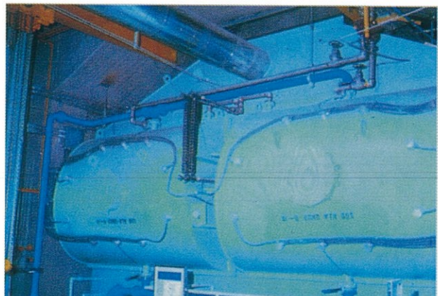
발전소용 연은합금 양극 설치모습 Installation View of Pb-Ag Anode on Power Plant Condenser
