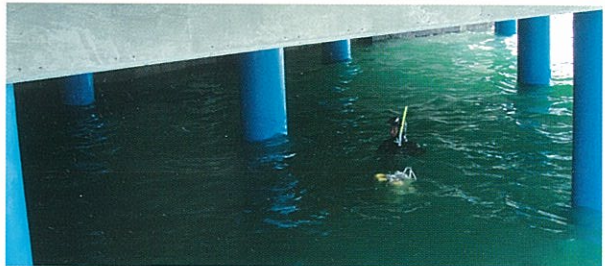
FRP 커버 설치/ Installation of FRP Cover
