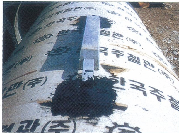
배관에 설치된 ZANODE / ZANODE Installed on Pipe
