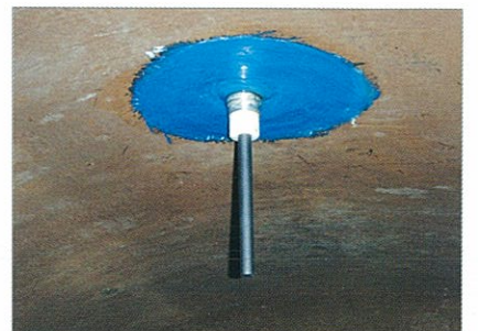
Installation View of M.M.O - Anode
