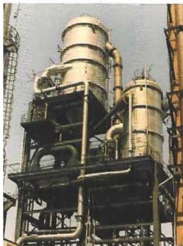
Ejector and Condensers in a urea plant.
