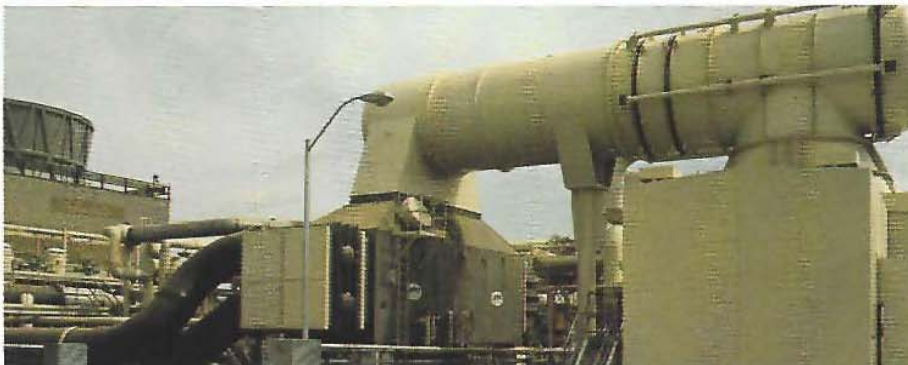
A 54,000 sq. ft. steam surface condenser for 32 MW geothermal power plant in California.
