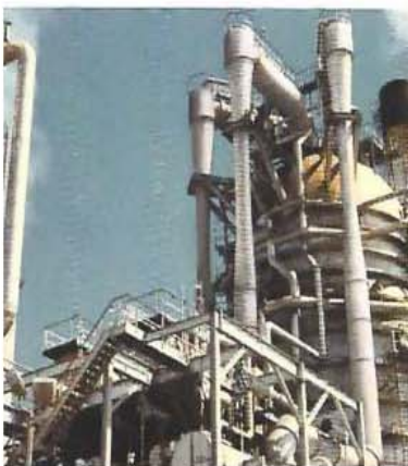
Triple element booster Ejectors in refinery service.
