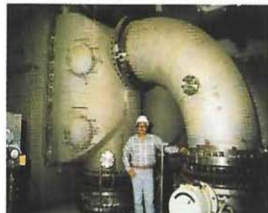
A 166,000 sq. ft. steam surface Condenser.
