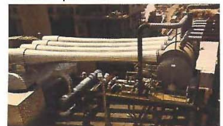
3,400 ton steam vacuum refrigeration unit.
