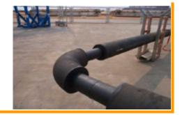
The Vikotherm insulative elastomer coating system is a development based on ordinary rubber technology.
