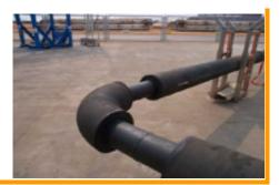
Flow assurance has become a critical aspect of deepwater developments. To protect subsea structures such as trees, manifolds and jumpers from hydrate formation they are insulated externally.
