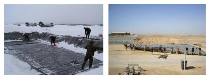
We manufacture tanks to internationally recognised military specifications, using commercial rubber coated textile options and PU materials for the tanks construction. These variations in construction materials allow the flexible tanks to be used in many other temporary storage applications for liquid chemicals and slurries.
